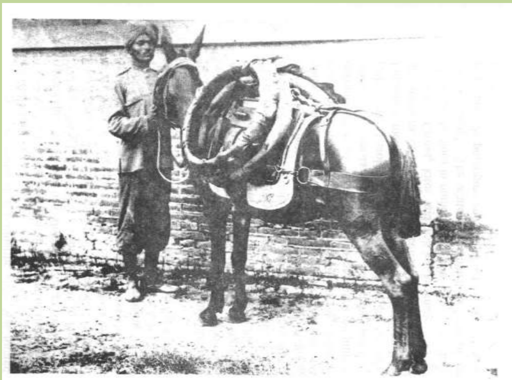
Telegraph wire in 40lb coils, with leather wrapping carried on an adapted mule-pack
